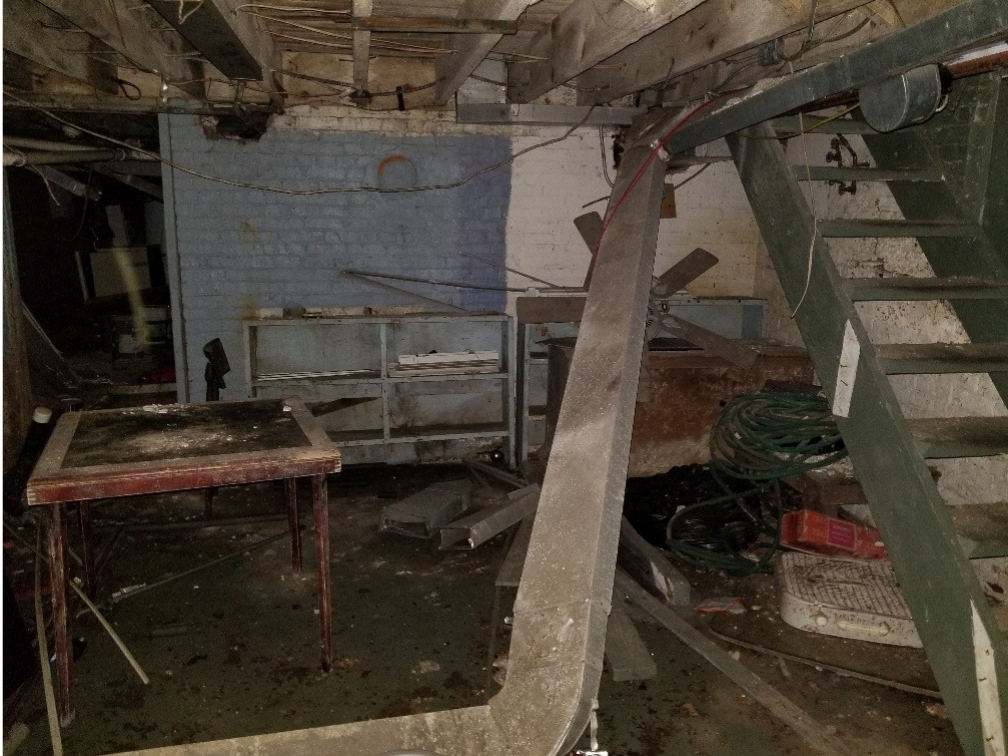
29. Cellar –Foundation walls and Floor framing still intact.
