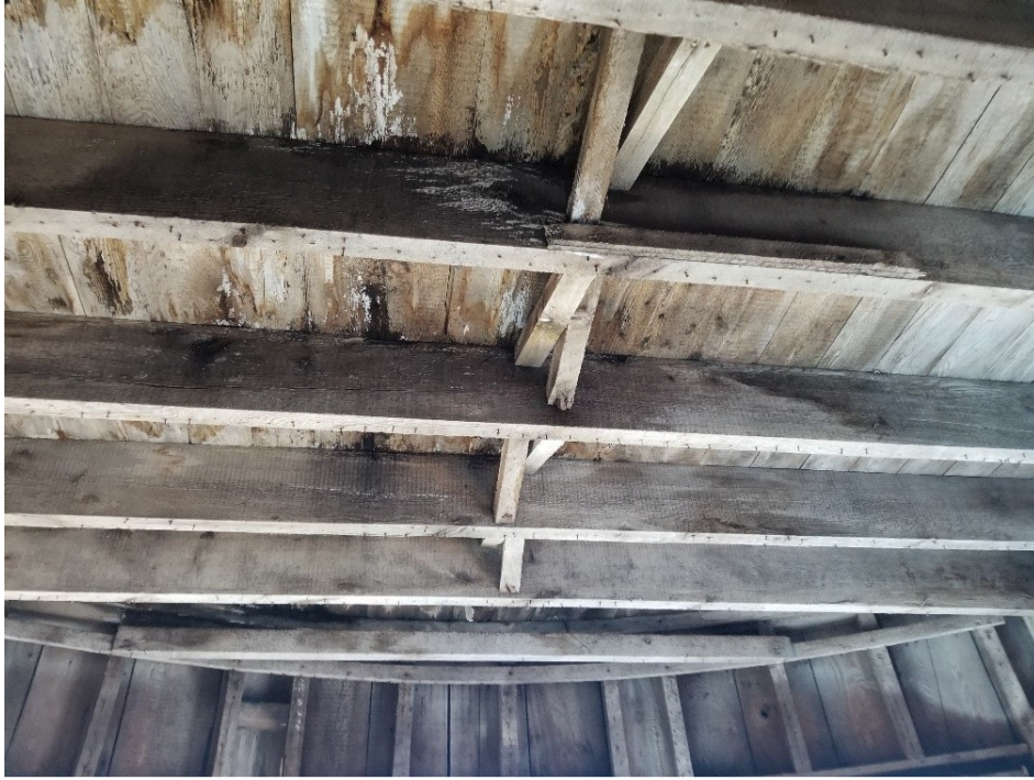
21. Second floor –Ceiling framing still intact.
