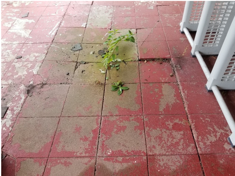
6. Exterior view –Floor at roofed terrace
