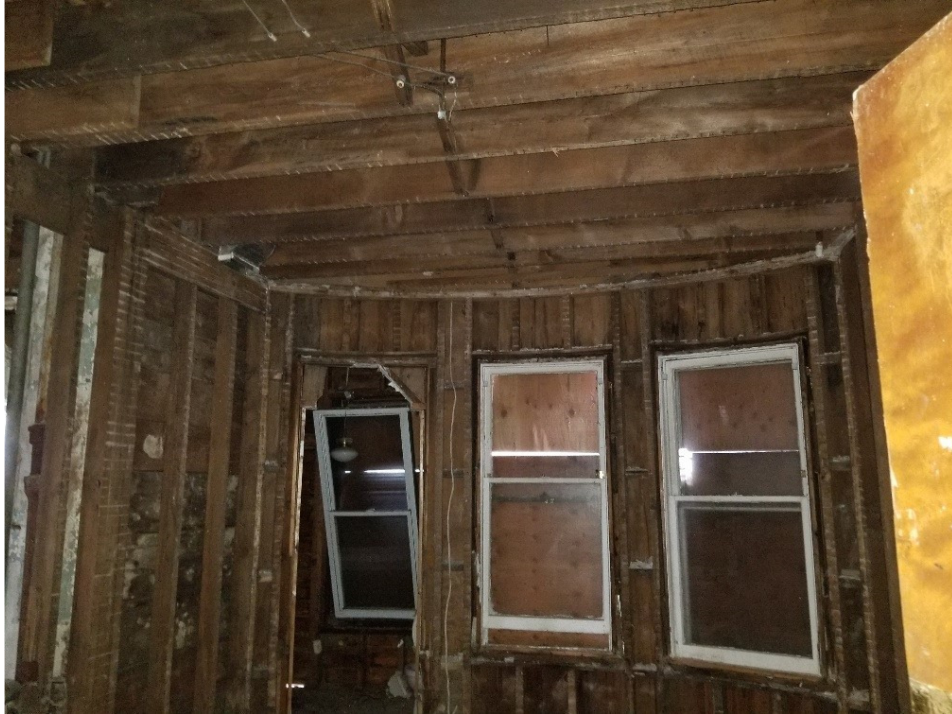
25. First floor –Portions, walls and ceiling framing still intact.
