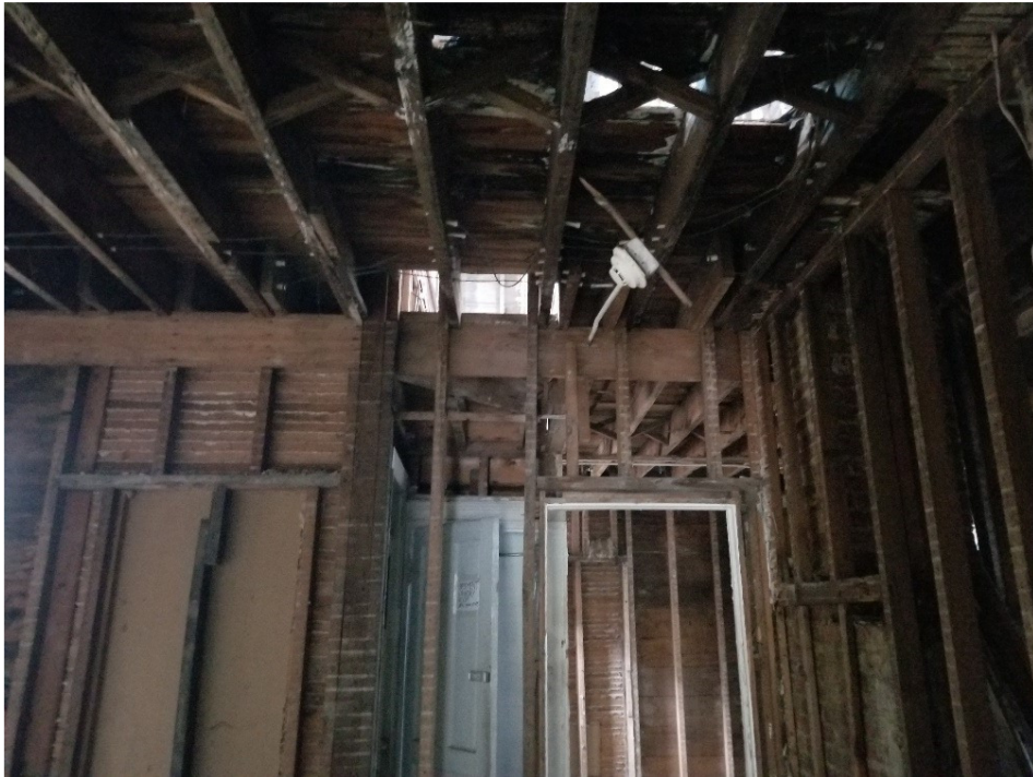
24. First floor –Portions, walls and ceiling framing still intact.
