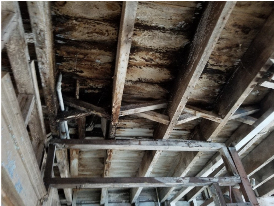
20. Second floor – Ceiling framing still intact.
