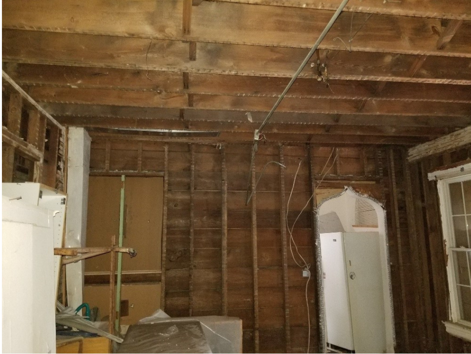
23. First floor –Portions, walls and ceiling framing still intact.
