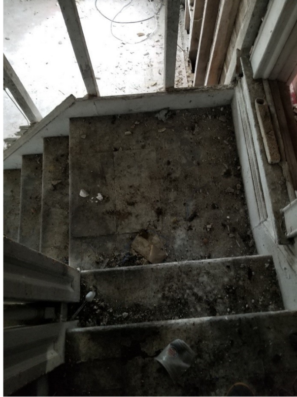
13. Attic floor –Stairs down to Second floor still intact.
