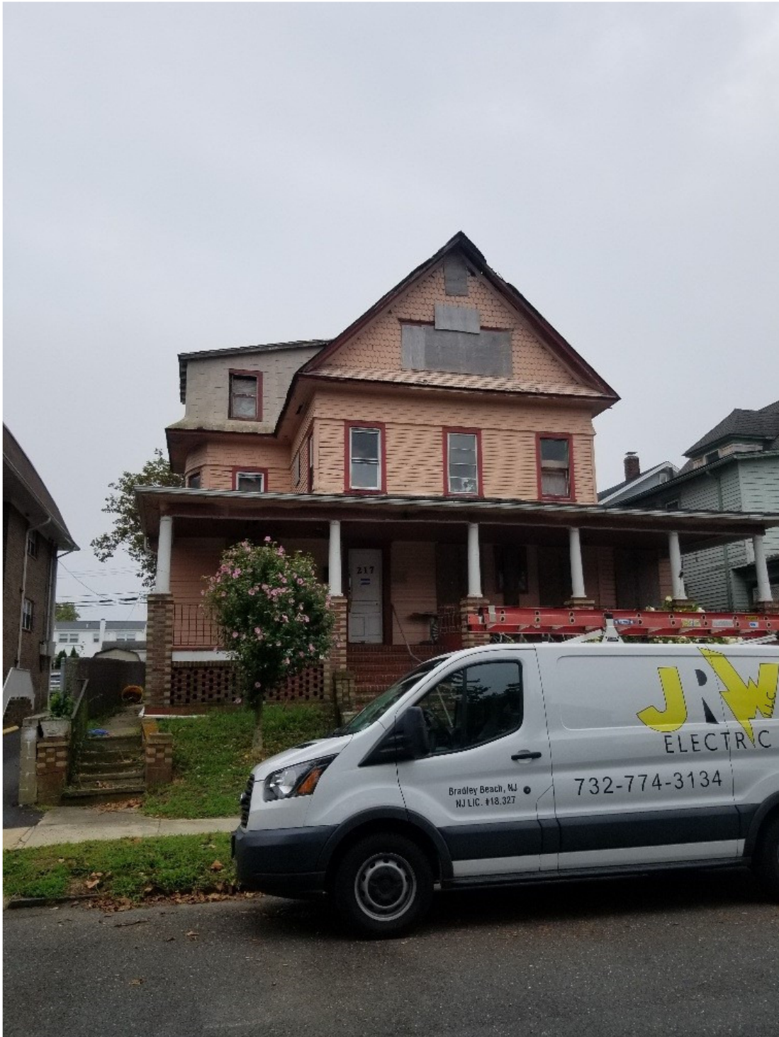
1. Exterior view –Front elevation
