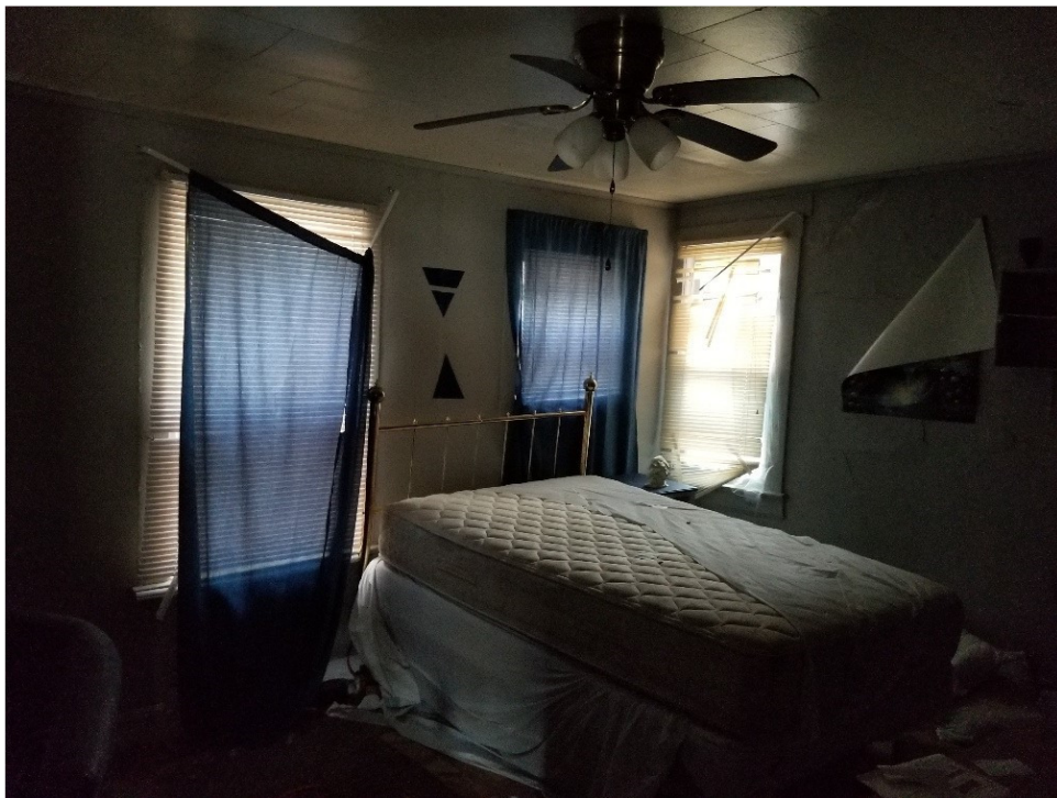
26. First floor –Some rooms sustain no damage at all.
