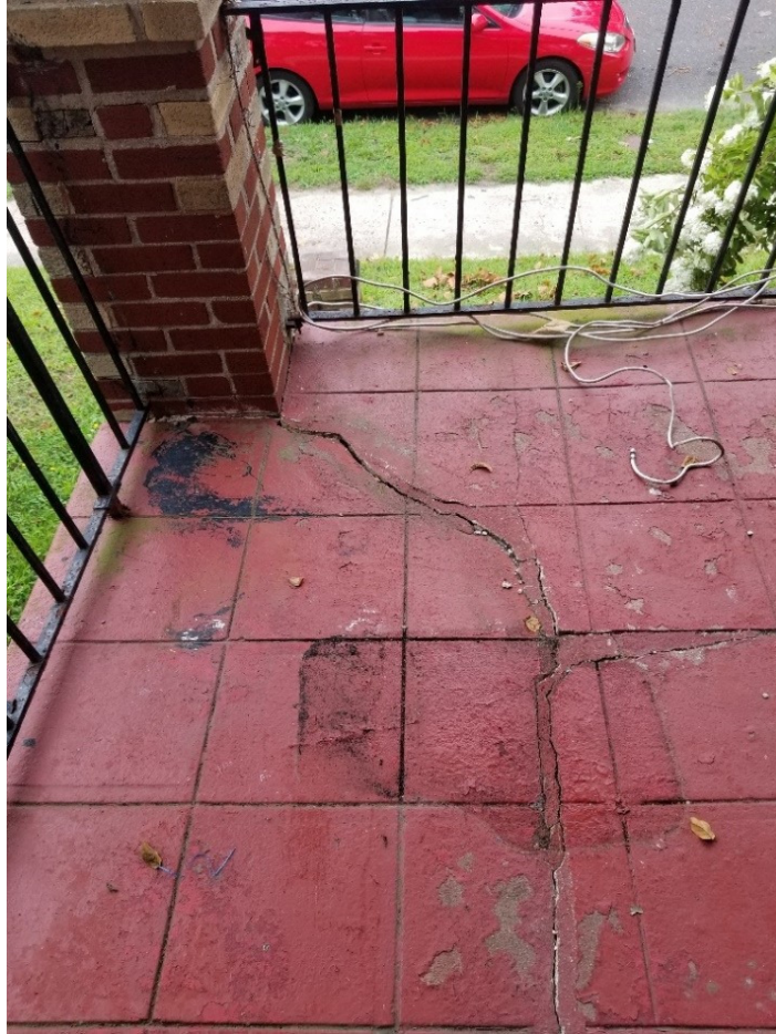
7. Exterior view –Floor at roofed terrace
