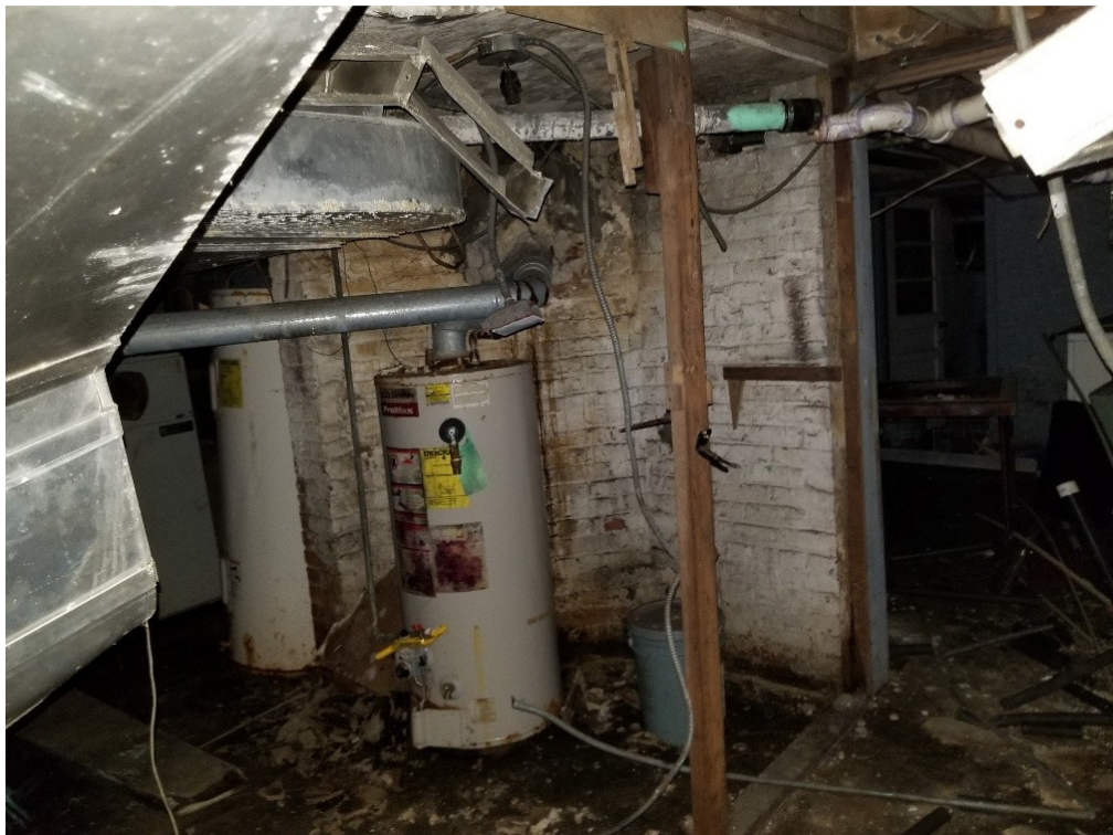
30. Cellar –Foundation walls and Floor framing still intact.
