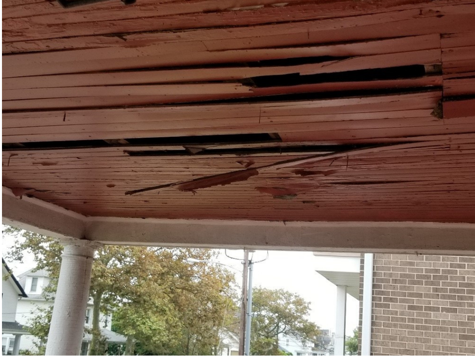
5. Exterior view –Ceiling at roofed terrace
