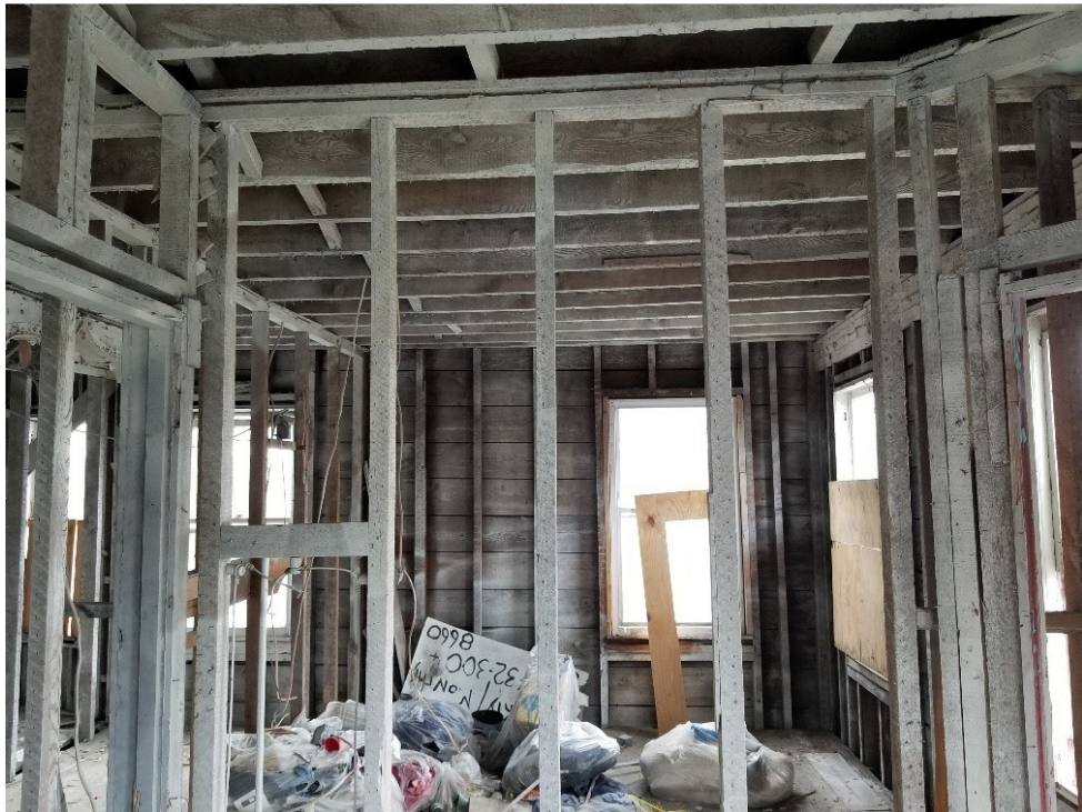
16. Second floor –Interior and exterior framing still intact.
