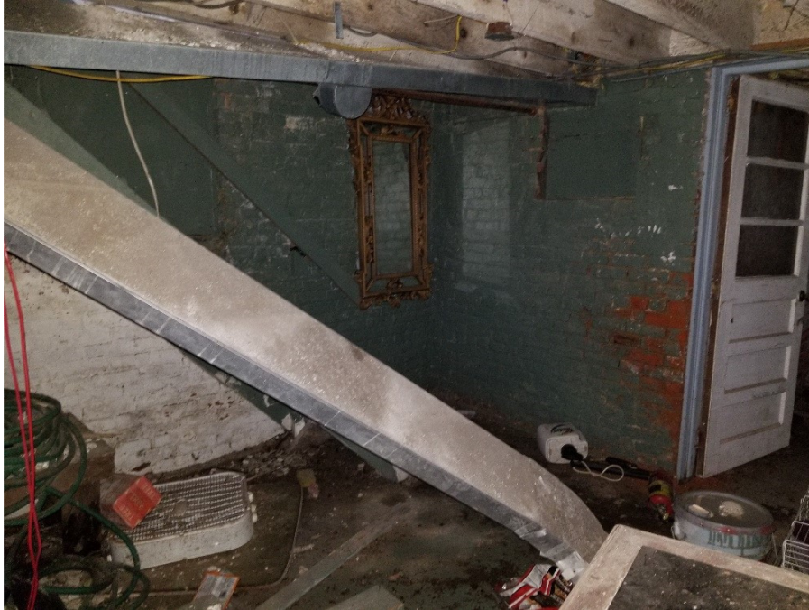
31. Cellar –Foundation walls and Floor framing still intact.
