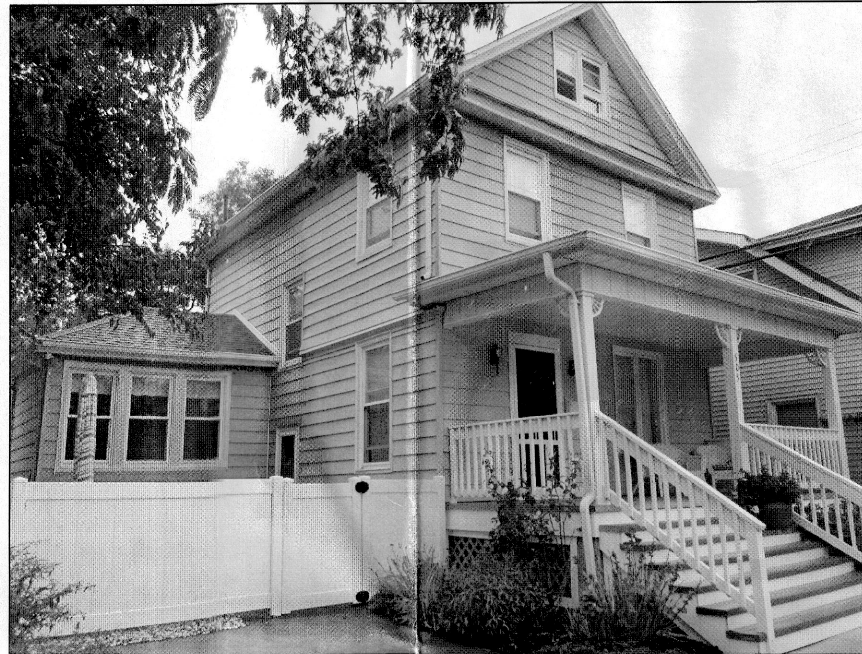
EXISTING CONDITIONS OF THE FRONT OF THE RESIDENCE
