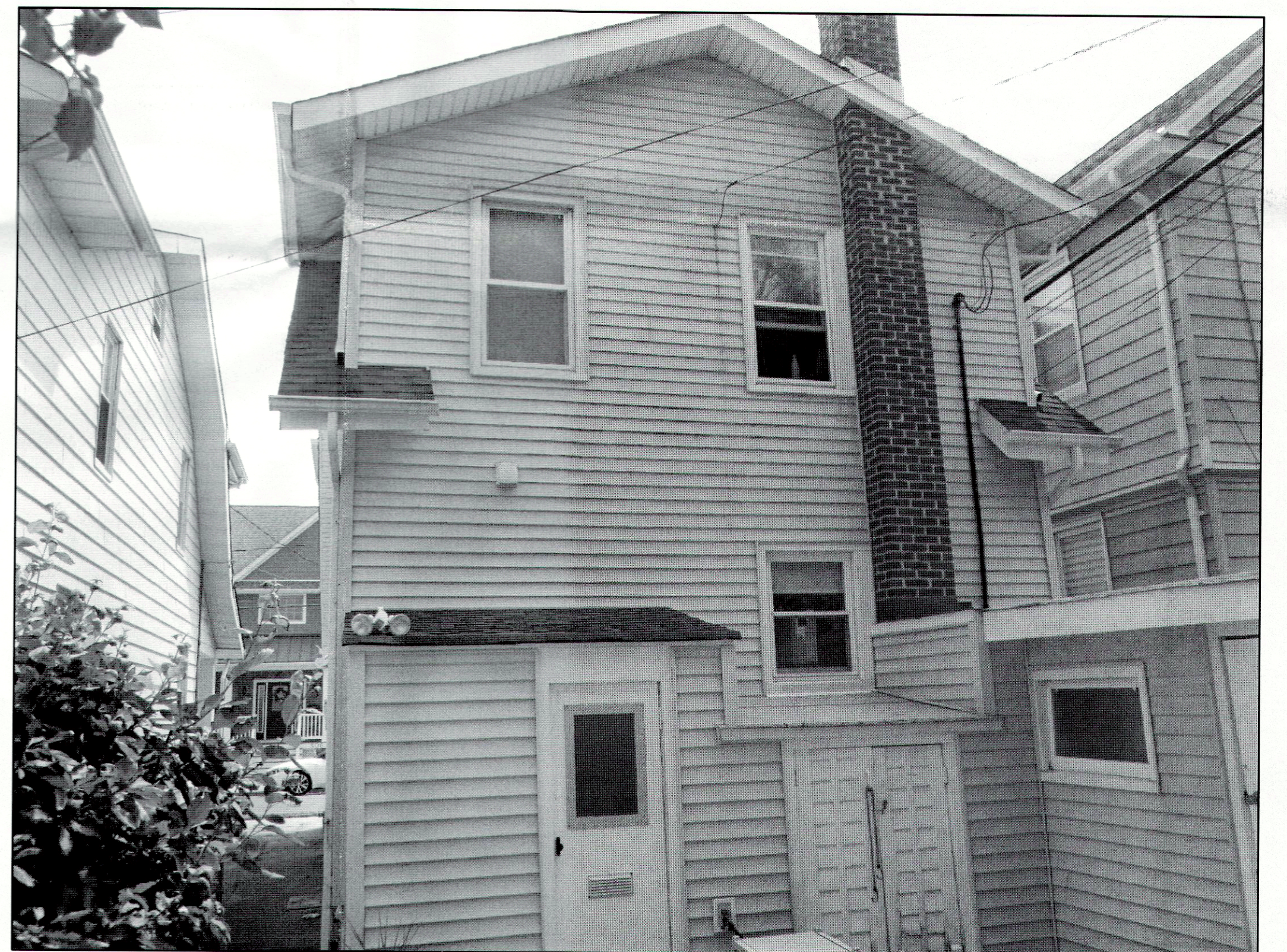
EXISTING CONDITIONS OF THE REAR OF THE RESIDENCE
