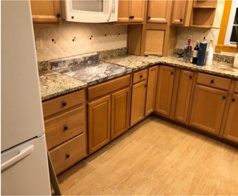
AFTER WET BAR (STOVE REMOVED AND CABINETRY/COUNTERS ADDED)
