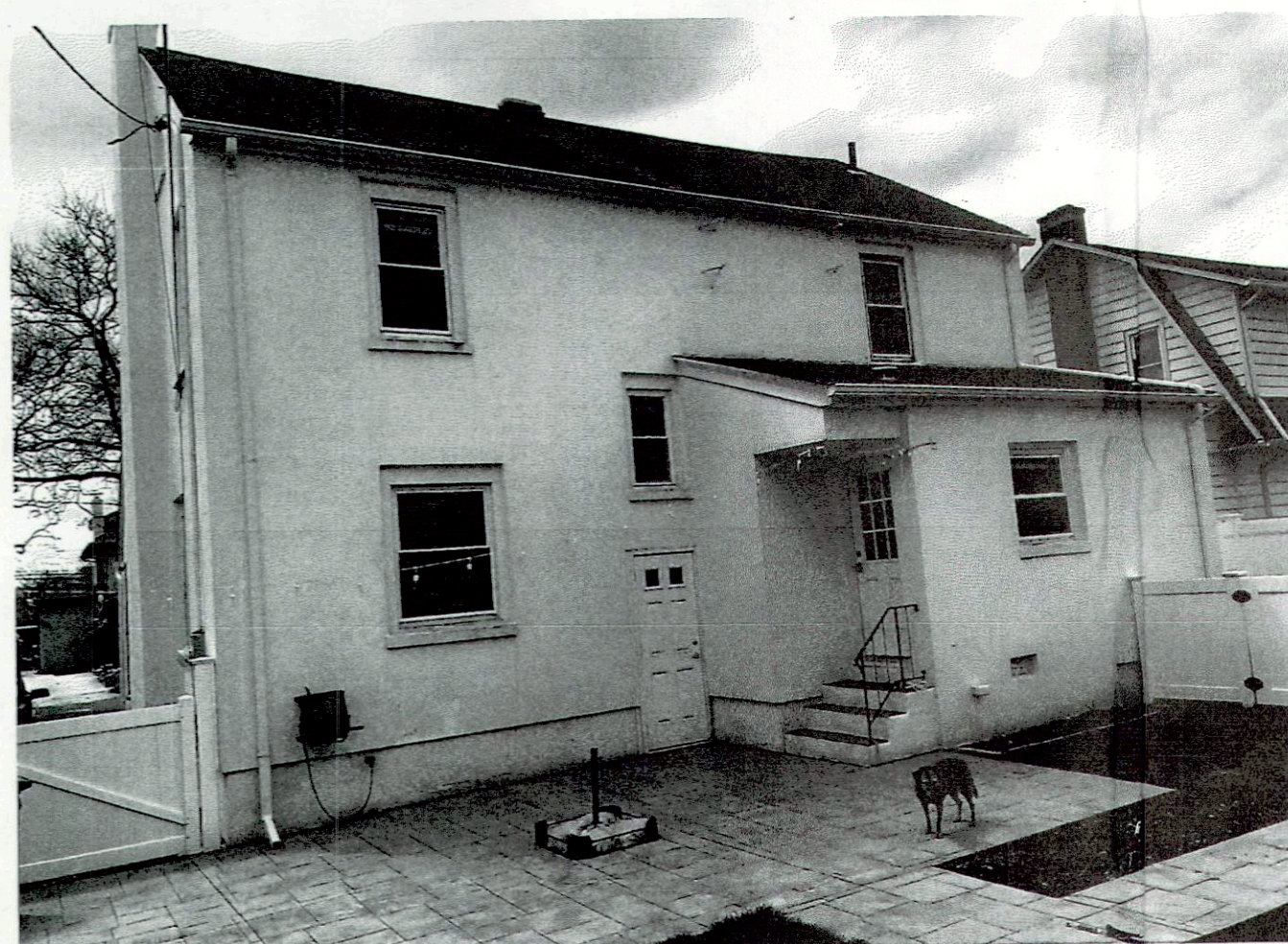
EXISTING CONDITIONS FROM NORTH EAST
