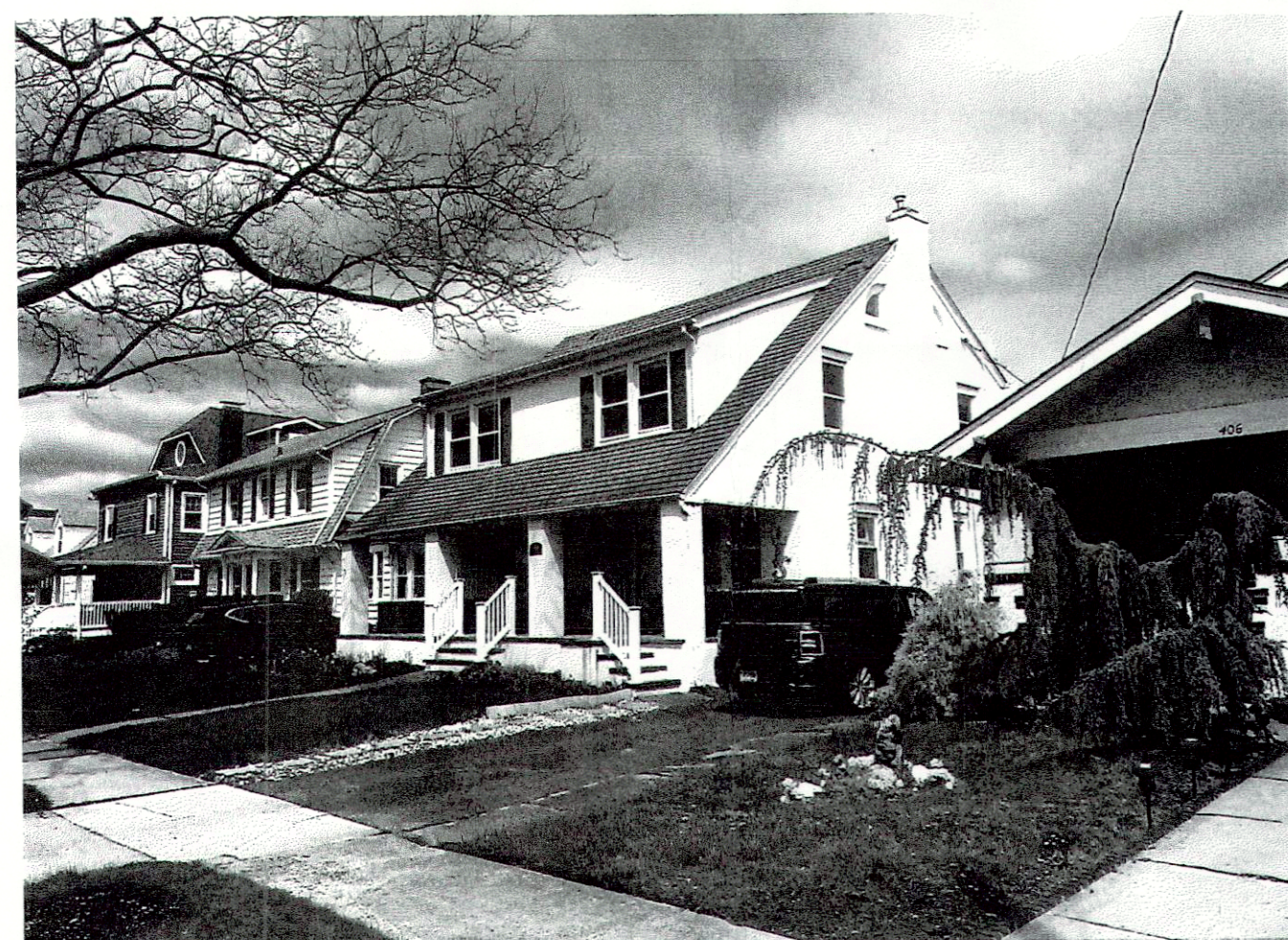
EXISTING CONDITIONS FROM SOUTH EAST
