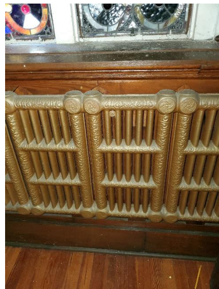
Image 8. Typical Sanctuary Decorative Radiator
